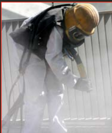
Conventional Grit Blasting
